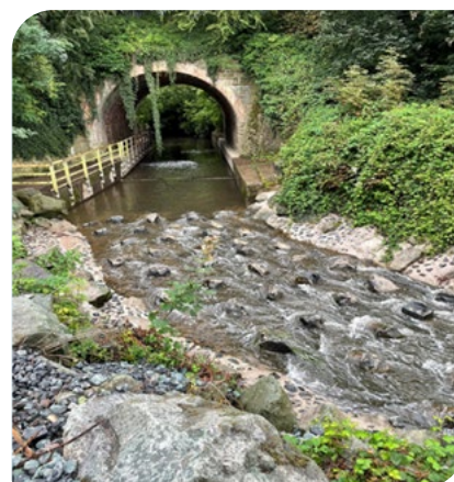
Kingfisher bridge, with fish barrier removed
